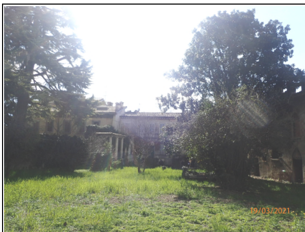
Figura 2.8: coperture in tegole in cotto
